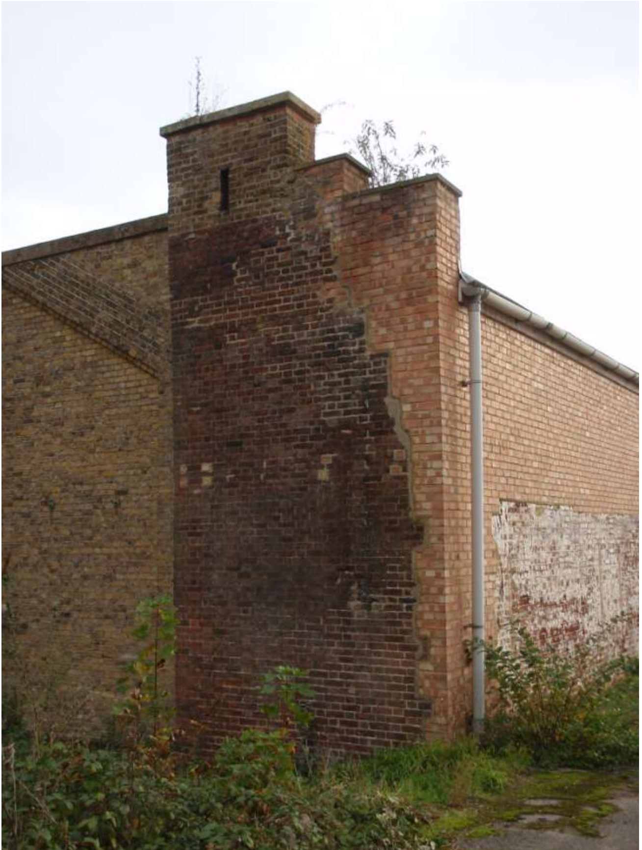
Plate 46. Detail of the rear of the Empty Case Store (left) showing butting on to remains of north end wall of Magazine 'A' (centre) and post-1960 repair to exposed wall following demolition of Magazine 'A' (right)
