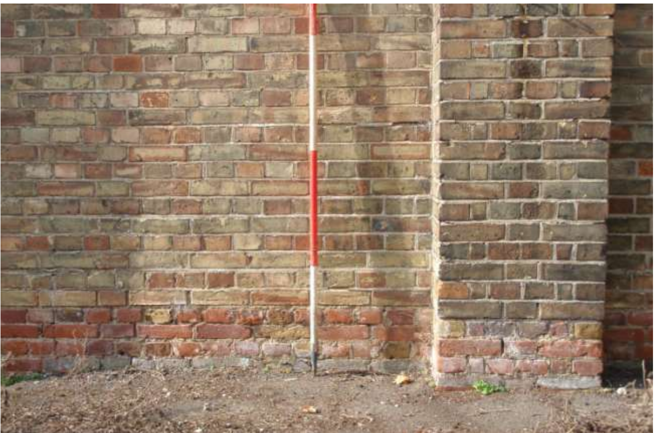
Plates 11,12. Inside face of boundary wall north of Main Gate. Note foundation courses-2m scale
