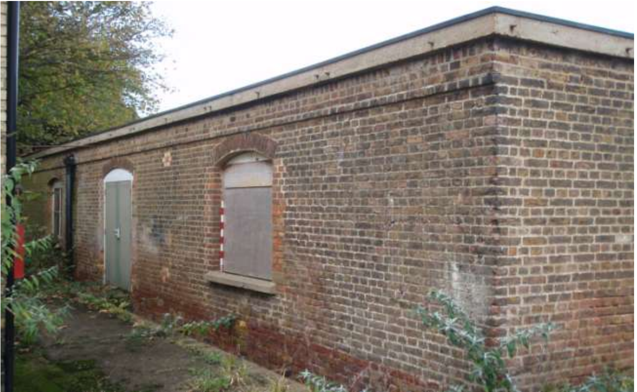
Plates 33,34. Small Arms Store showing rebuilt window opening and modern concrete flat roof-1m scale
