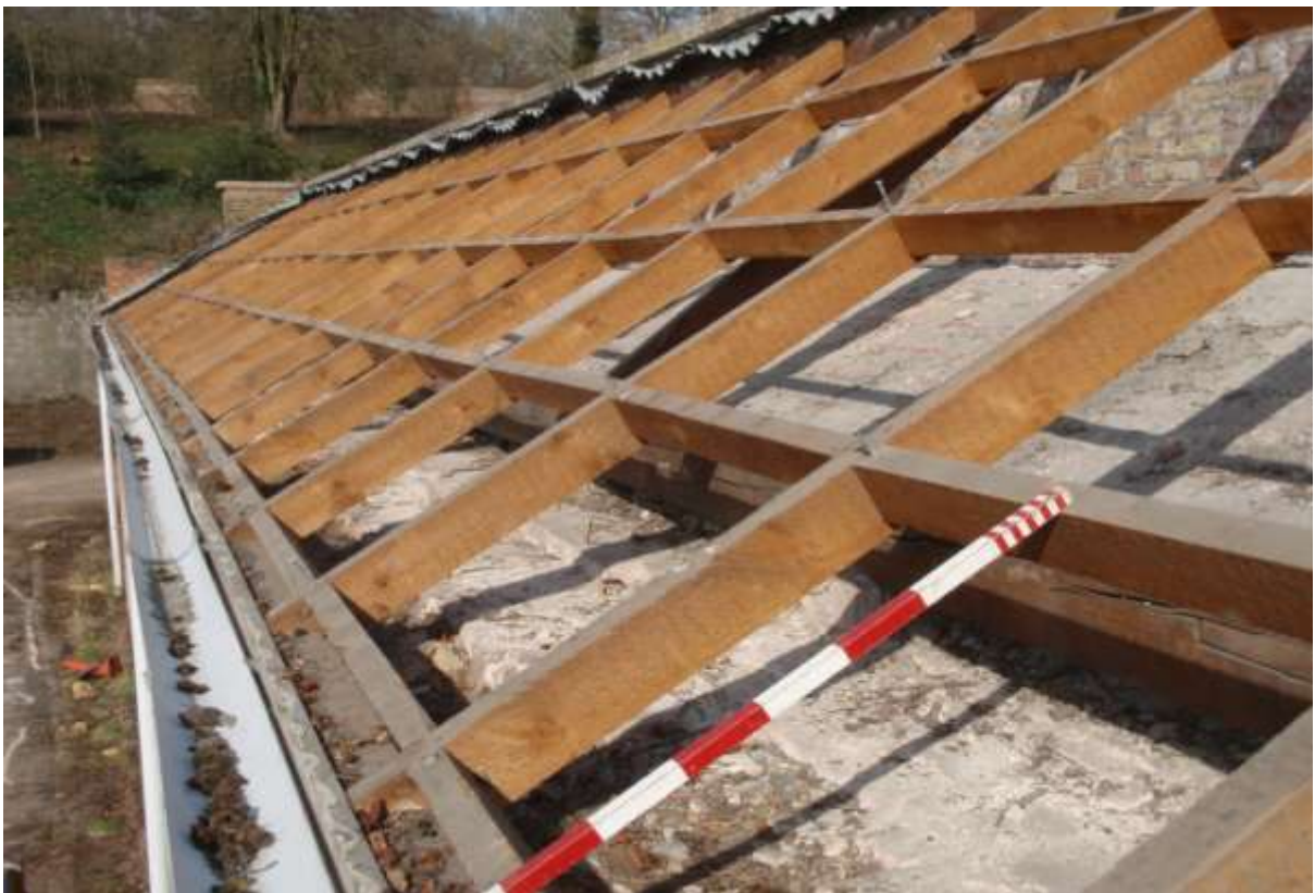
Plate 80. Removal of the corrugated roof exposed the 1811 brickwork
