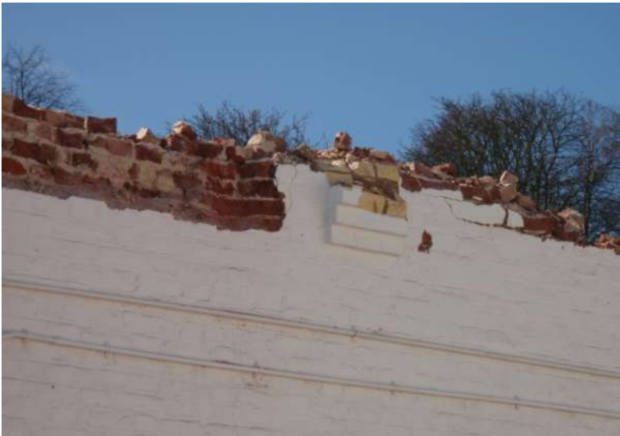
Plate 82. Showing the inserted corbelled brick brackets
