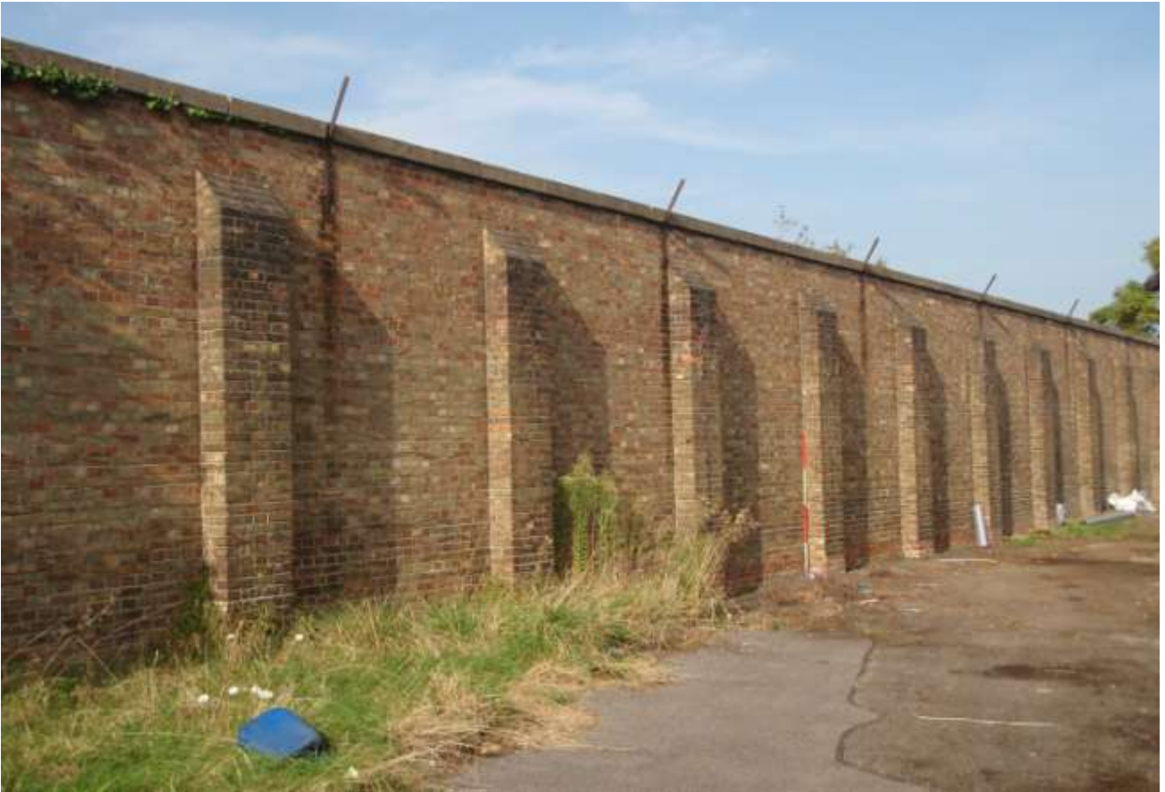
Plates 11,12. Inside face of boundary wall north of Main Gate. Note foundation courses-2m scale
