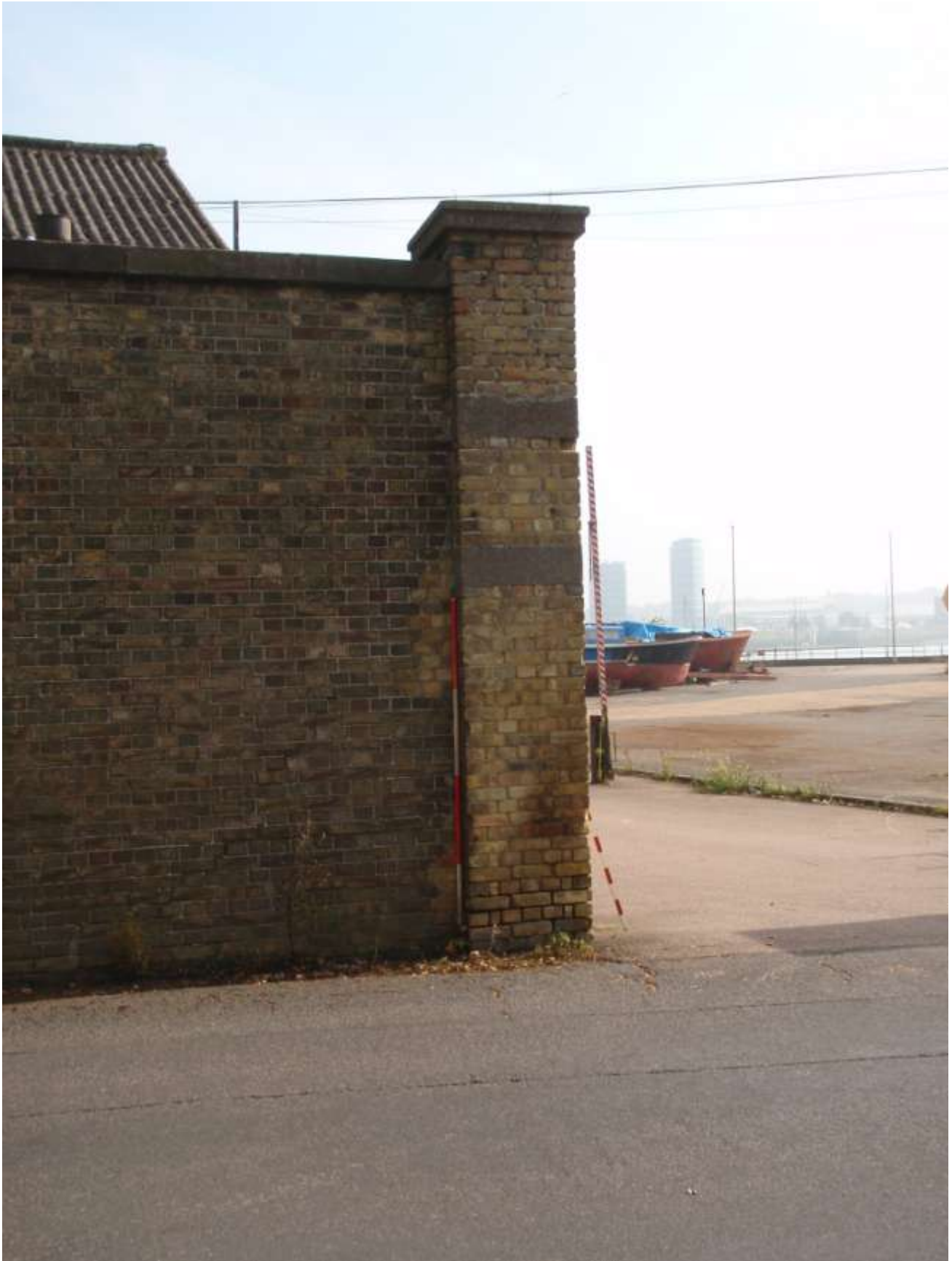
Plate 8. Later phase gate pillar in yellow stock brick keyed into earlier build wall -2m scale
