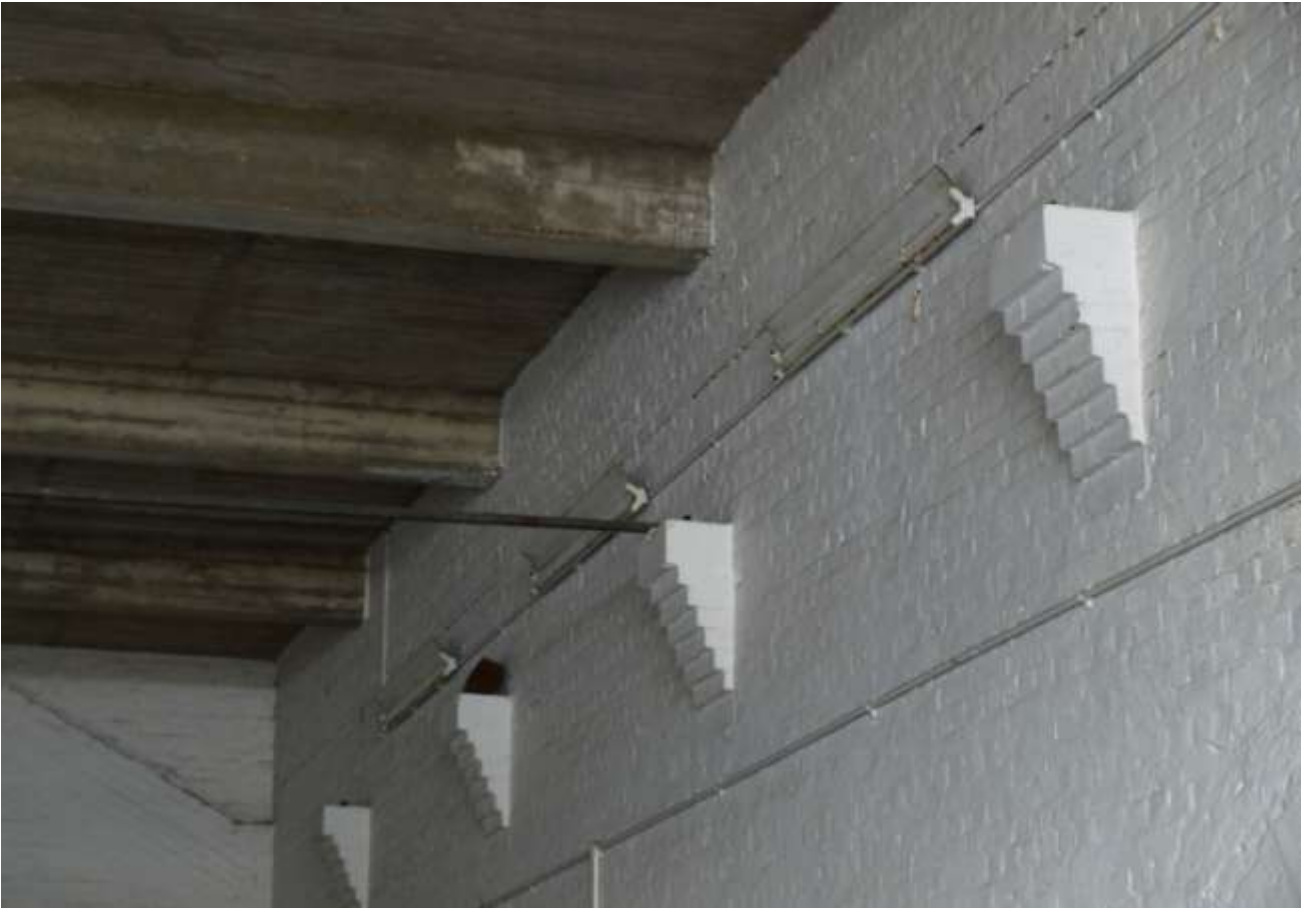
Plates 64, 65. Showing brick corbelling for original 1893 roof and (below) replacement concrete roof
