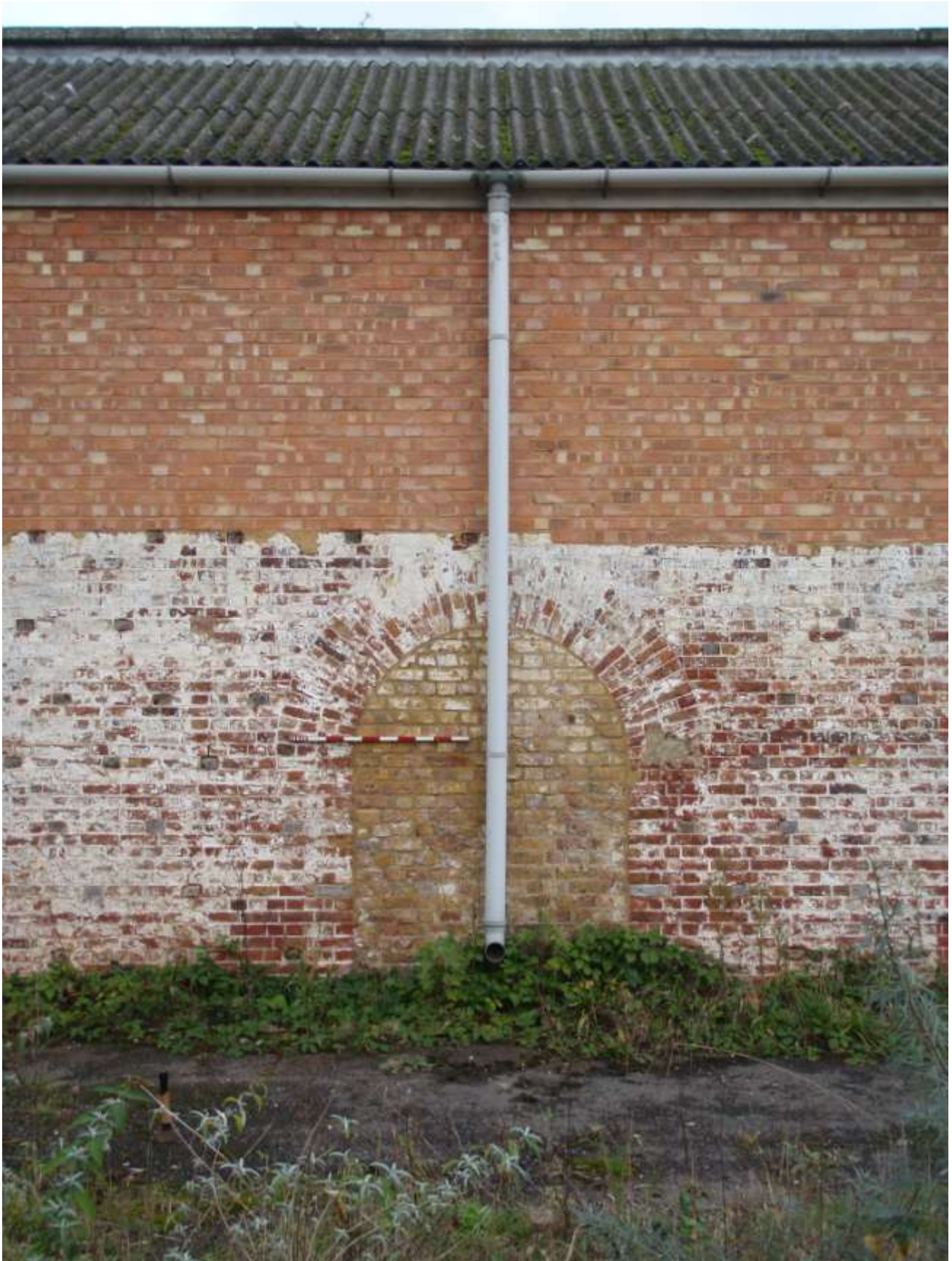
Plate 49. Showing the internal face of the north wall of Magazine 'A' with the entrance blocked with yellow stock bricks. Following demolition in post-1960 the wall has been rebuilt with fletton bricks-1m scale
