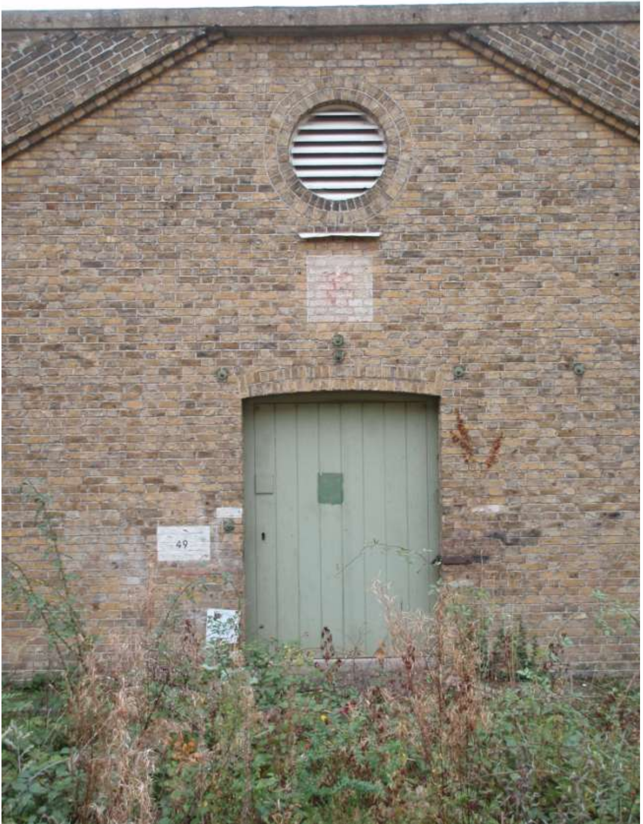
Plate 48. Rear wall of the 1893 Empty Case Store showing the original build
