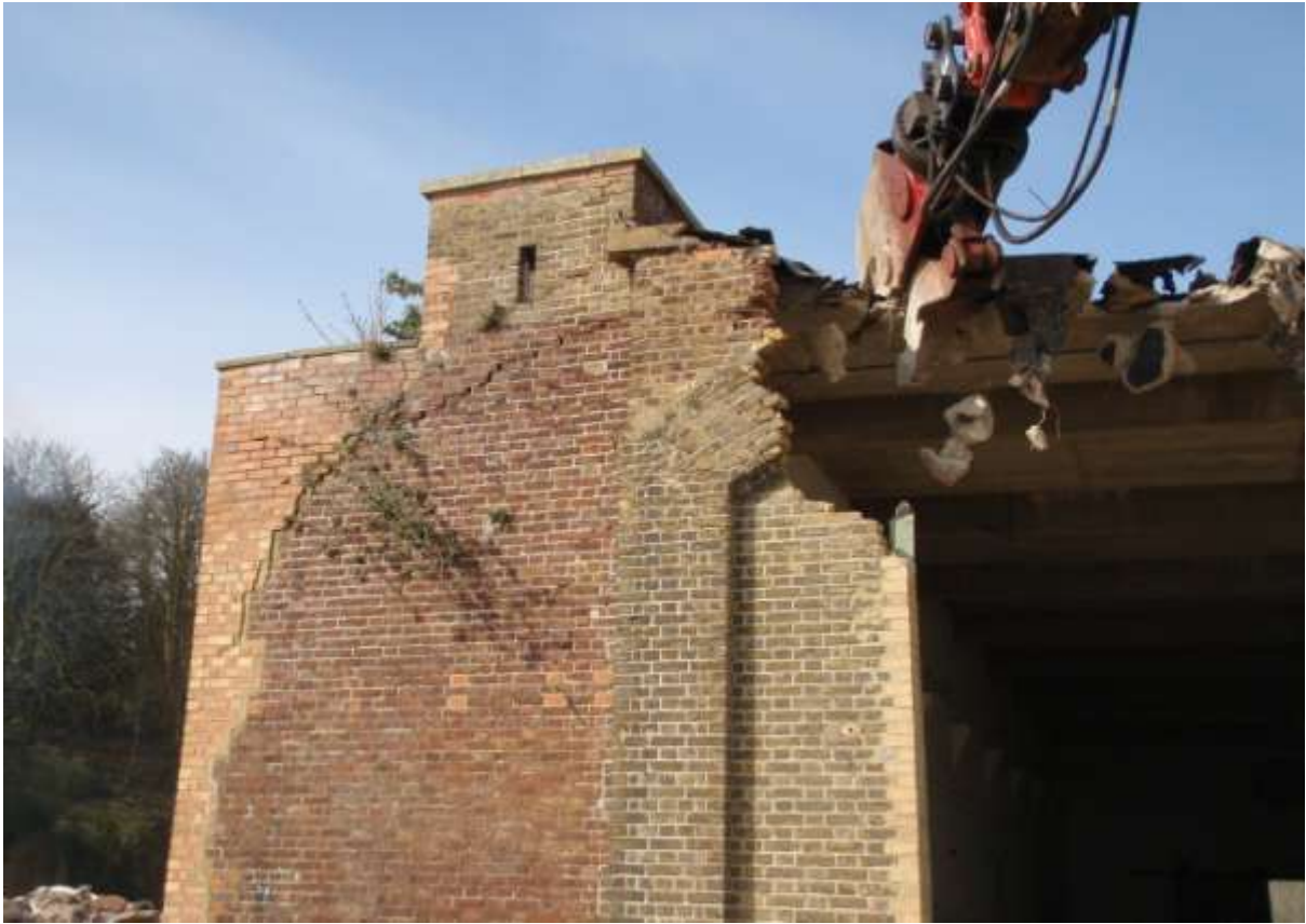
Plate 79 Phases of brickwork
