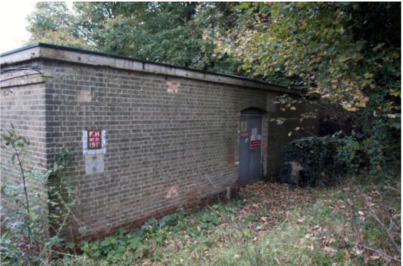
Plates 33,34. Small Arms Store showing rebuilt window opening and modern concrete flat roof-1m scale
