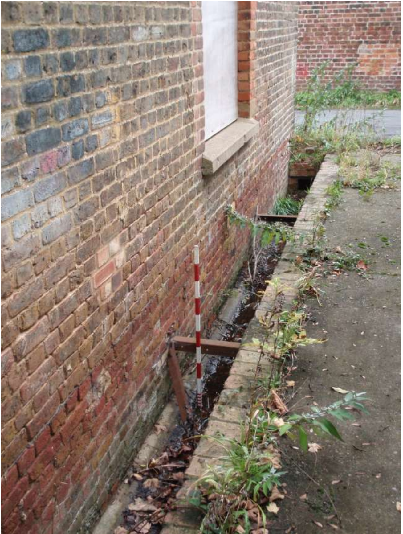
Plate 37. Small Arms Store showing drainage gully, foundation bricks and damp course- 1m scale
