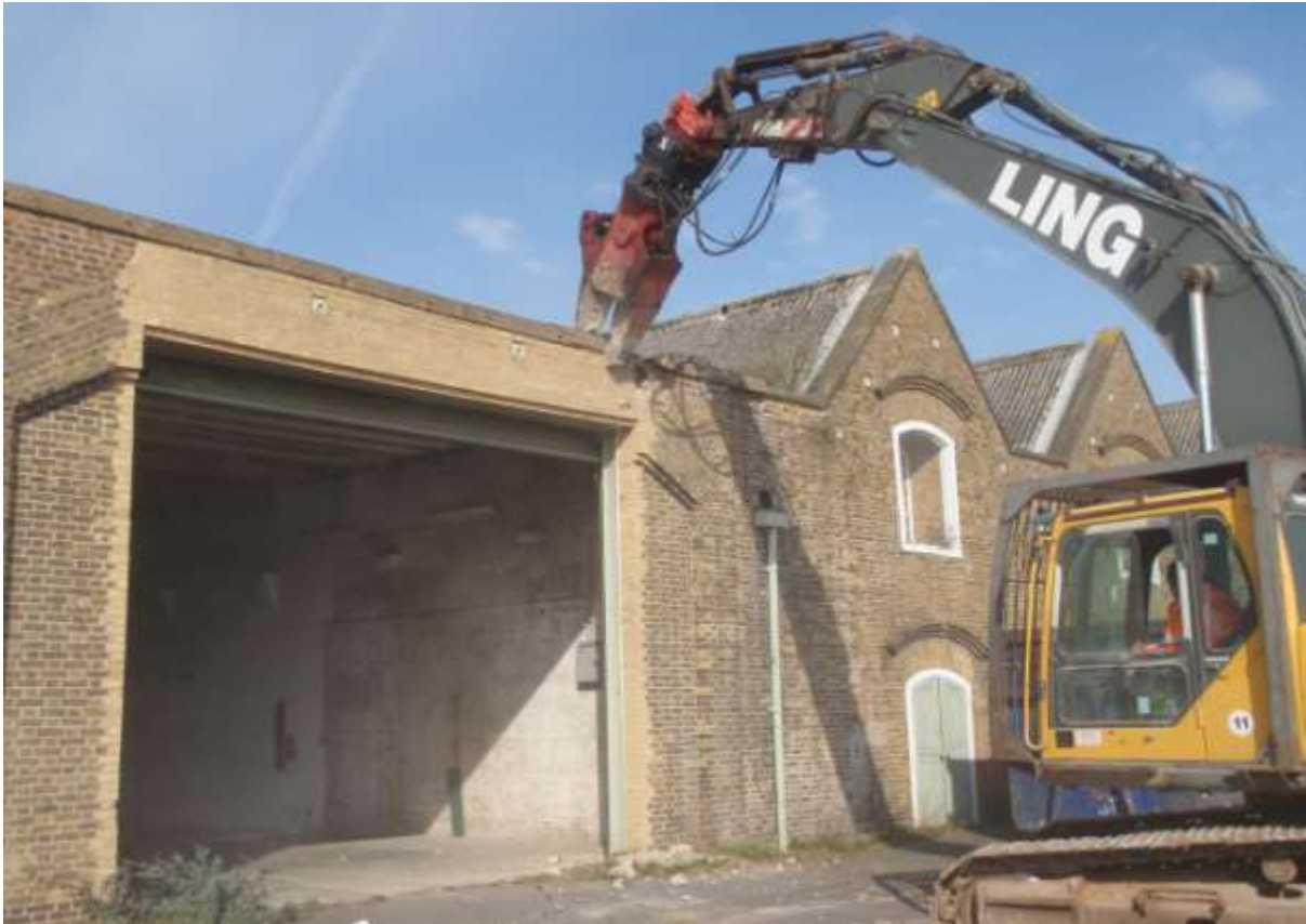
Plate 77. Demolition of the Empty Case Store
