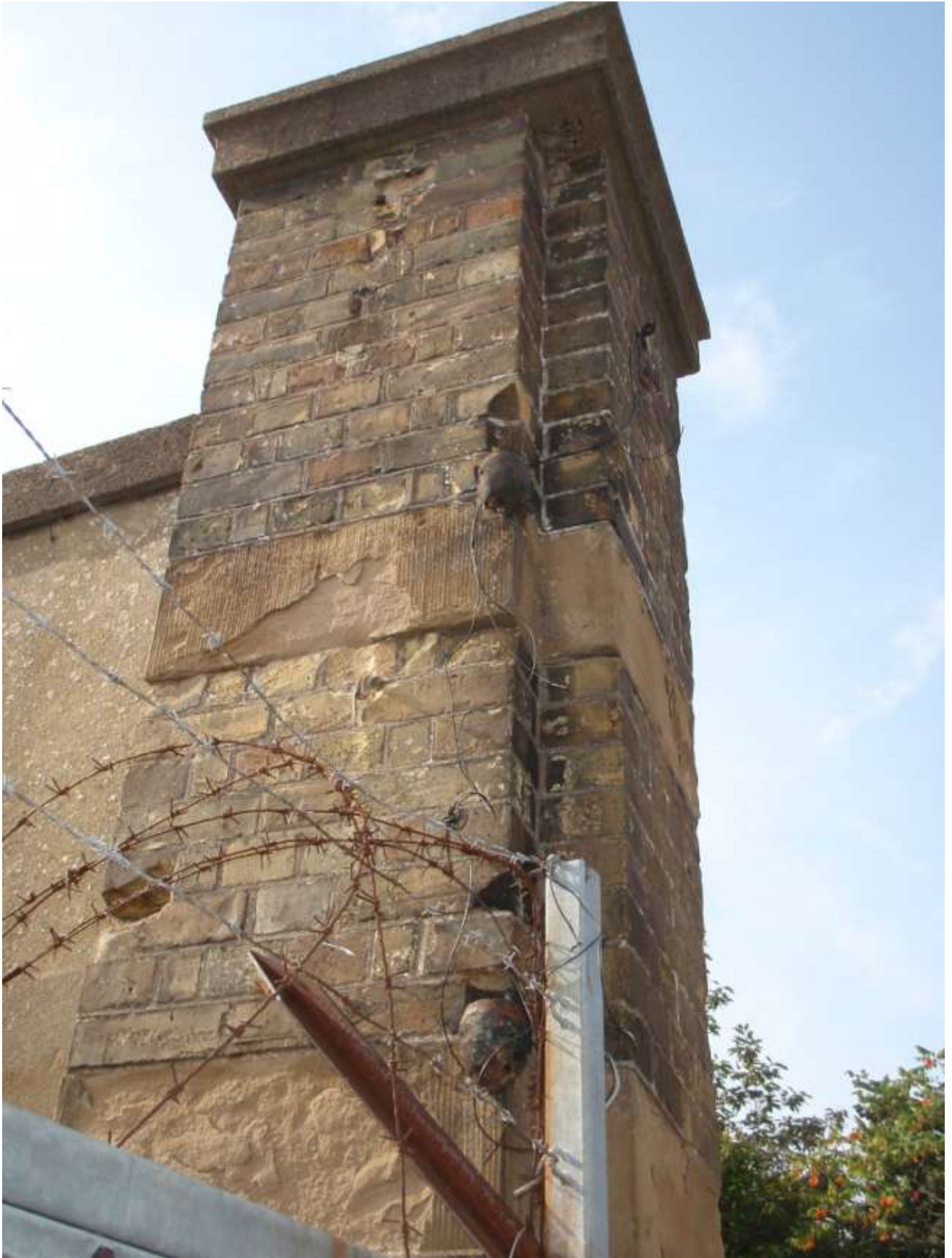
Plate 7. Detail of 'sandstone' pillar. Note pintles for the original gate
