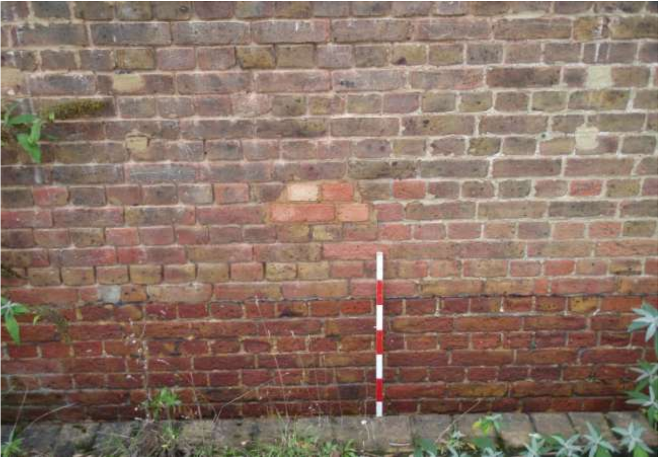
Plates 38, 39. Small Arms Store showing damp course and (below) internal view of concrete roof-1m scale
