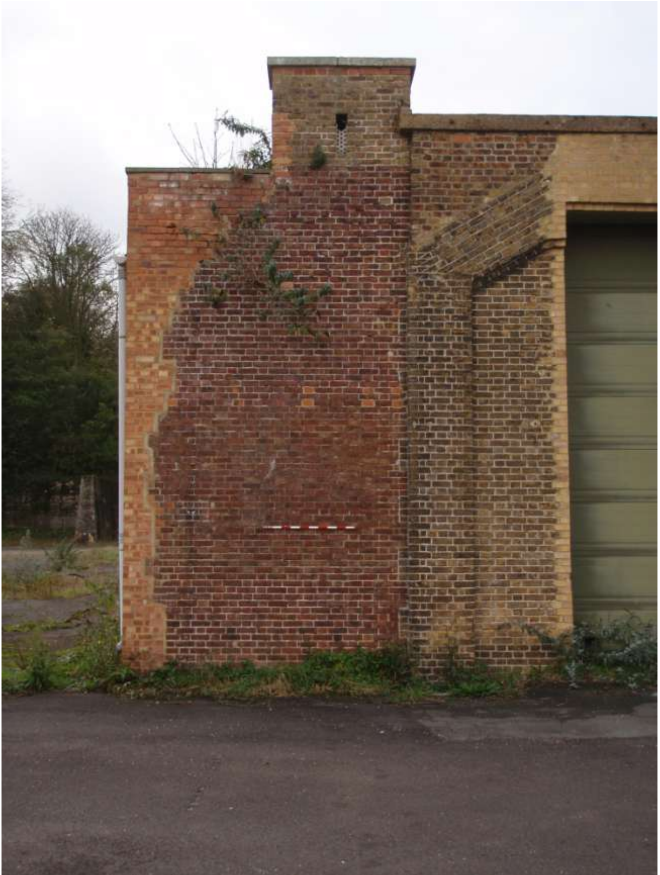
Plate 47. Detail of the front of the Empty Case Store (right) showing butting on to remains of north end wall of Magazine 'A' (centre) and post-1960 repair to exposed wall following demolition of Magazine 'A' (left)
