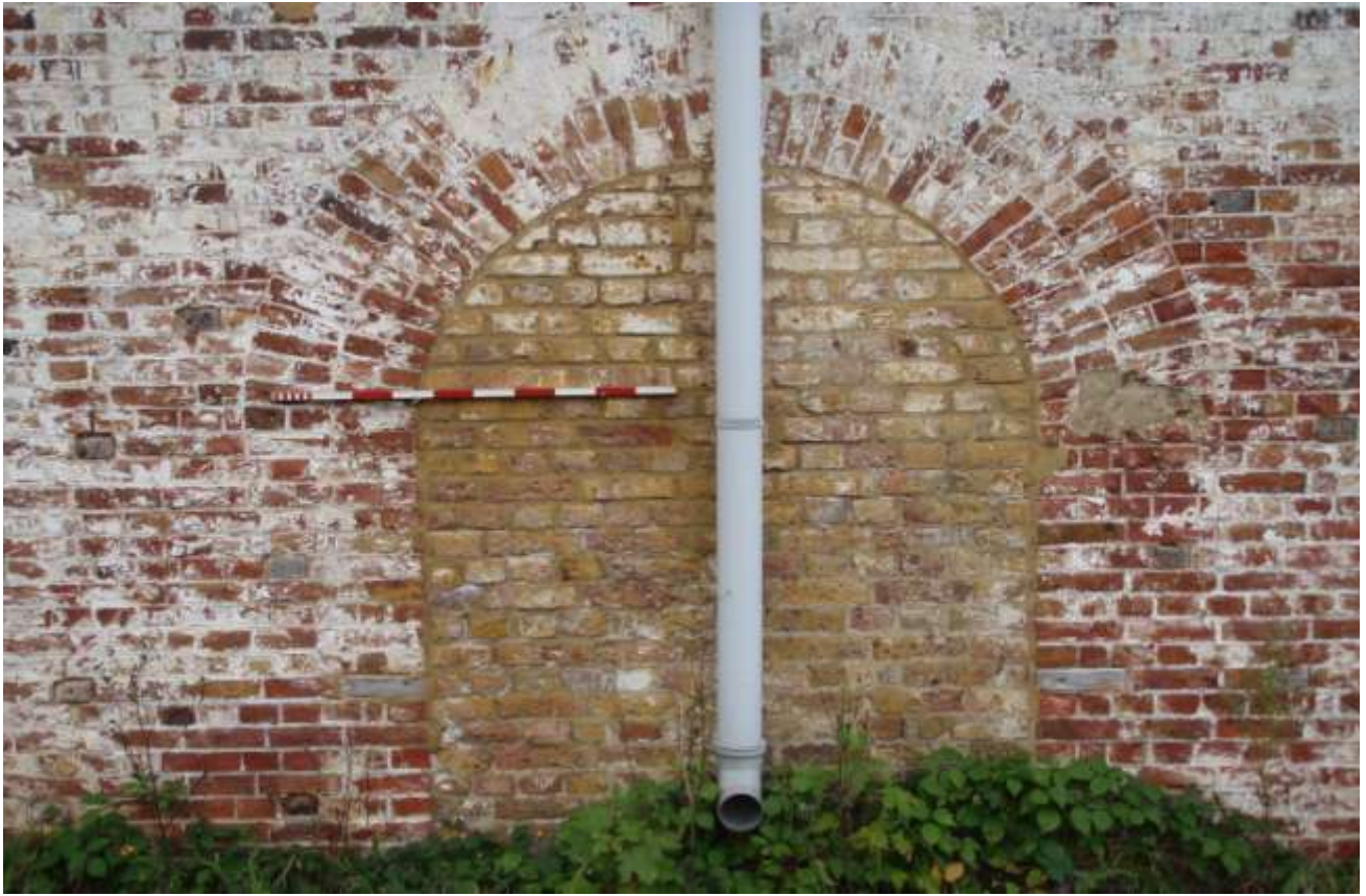
Plates 51, 52, Detail of arch and (below) blocked ventilation slots in the wall of Magazine 'A' -1m scale
