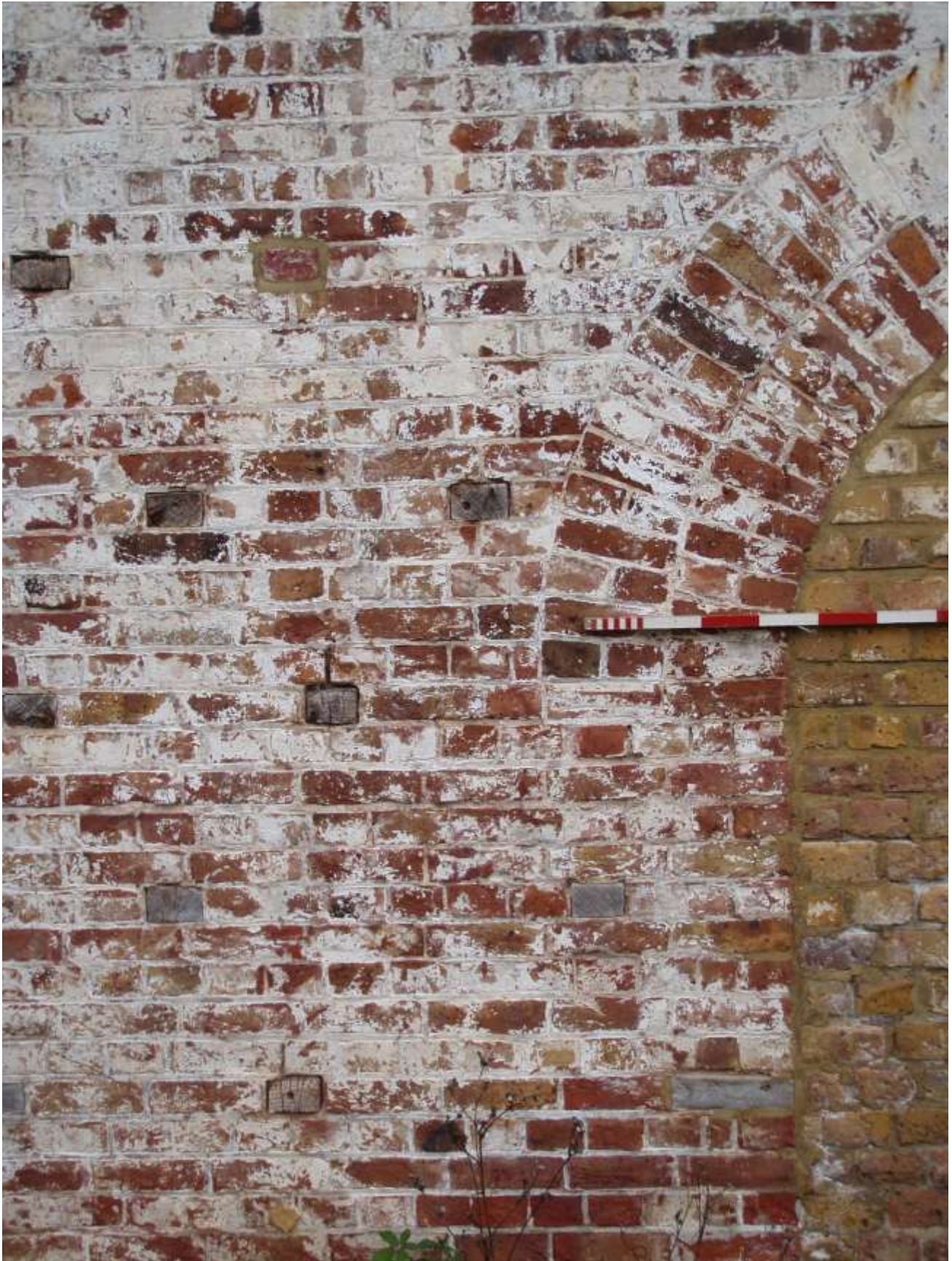
Plate 50. Detail of the internal wall of Magazine 'A' showing hardwood blocks in the brickwork to facilitate fixing internal panelling- 1m scale (10cm segments)
