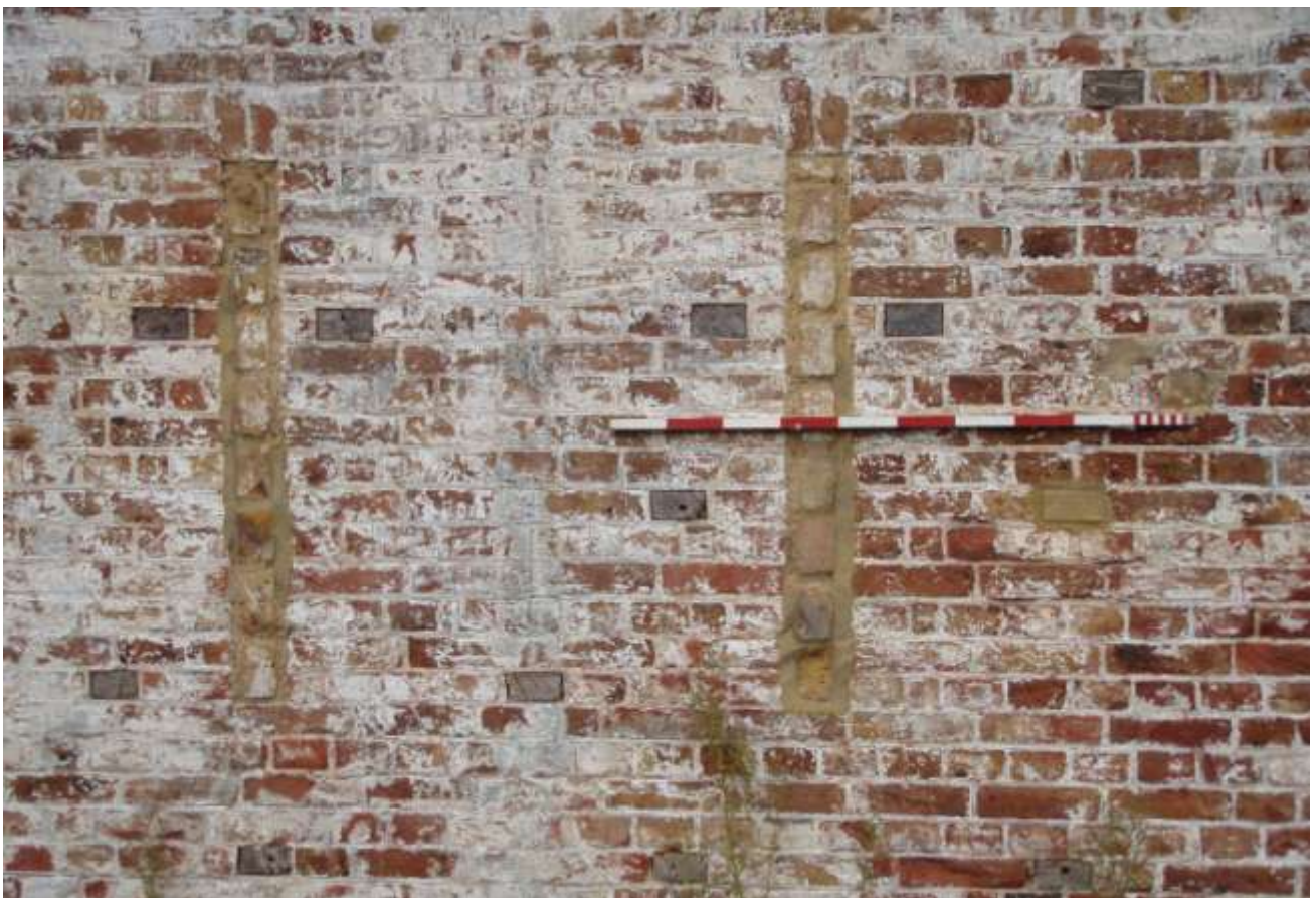
Plates 51, 52, Detail of arch and (below) blocked ventilation slots in the wall of Magazine 'A' -1m scale
