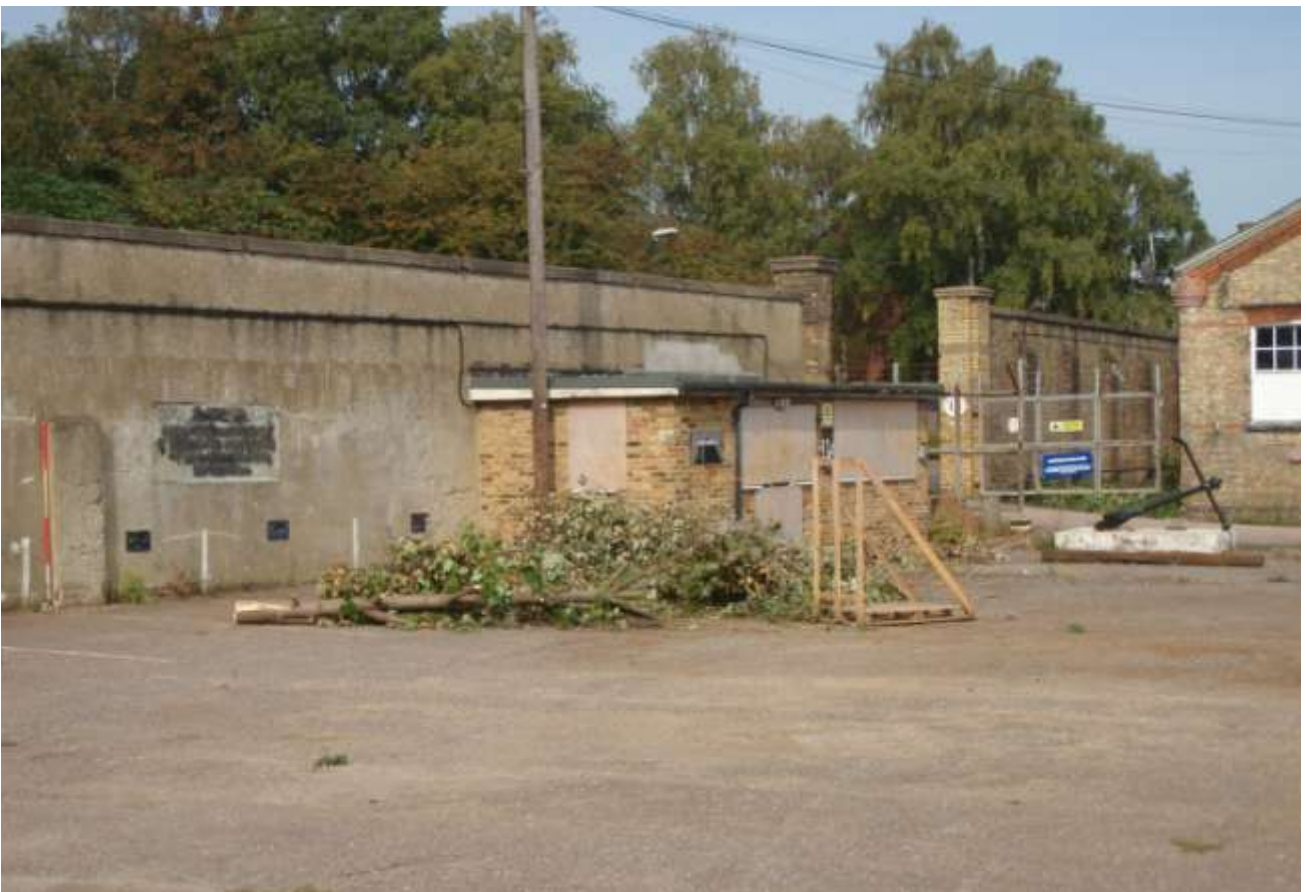
Plates 9,10. Main Gate looking out. Note concrete render to internal face of south wall
