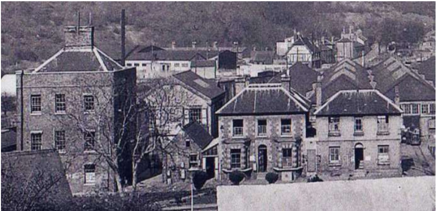
Figure 40. A view to the North over the roofs of the No. 3 Shell Store and the Wet Guncotton Store to the civilian houses turned after purchase into Offices. Beyond can be seen the roof and entrance of the Filled Shell Store
