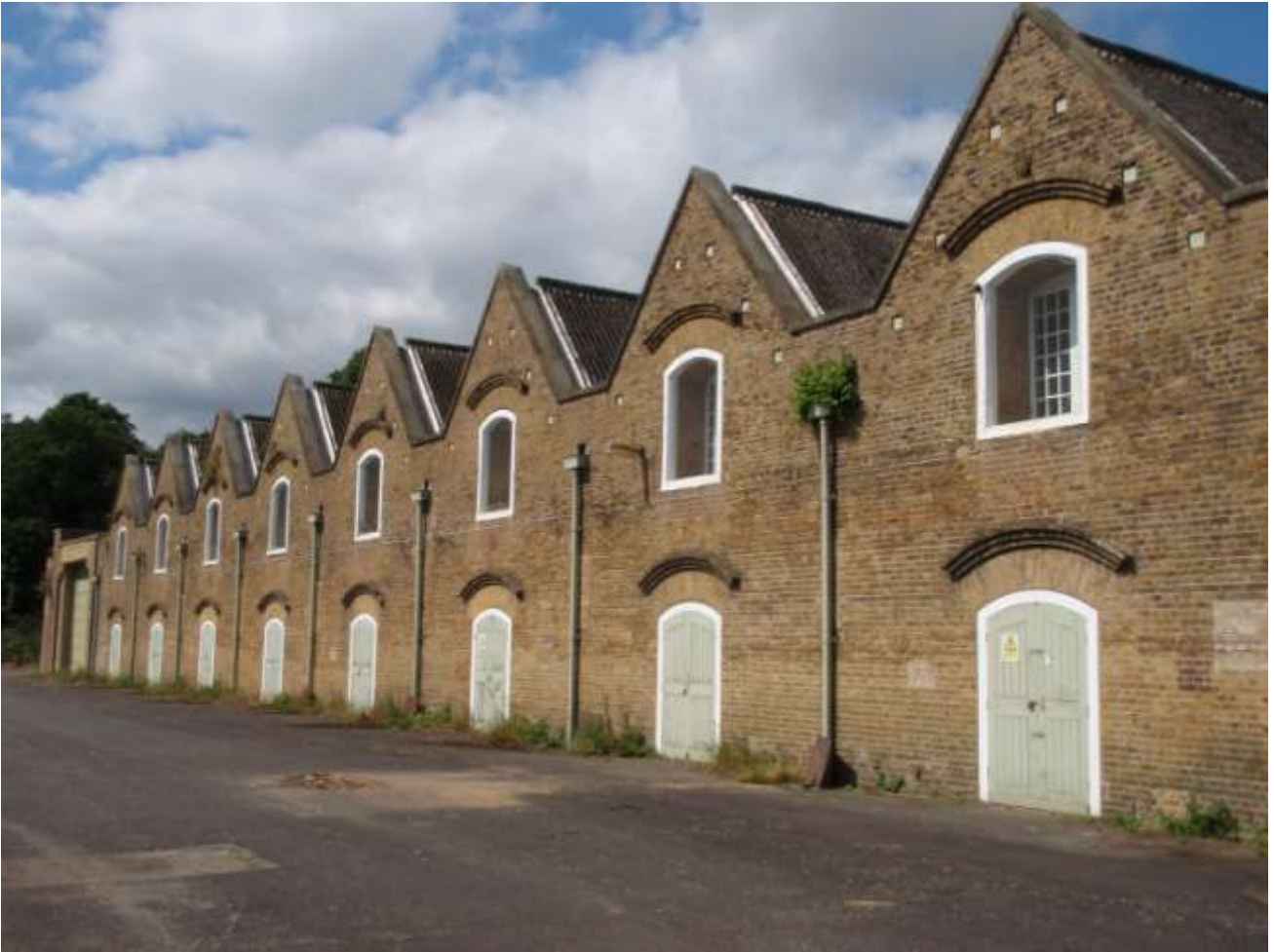
Plate 68. Front view of Magazine 'B' built by 1857 (looking SW)
