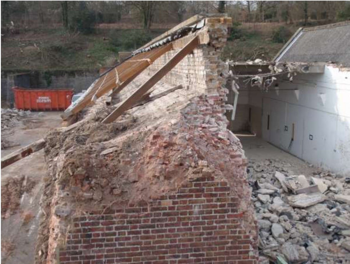
Plate 81. The sloped brickwork upper surface of Magazine 'A'
