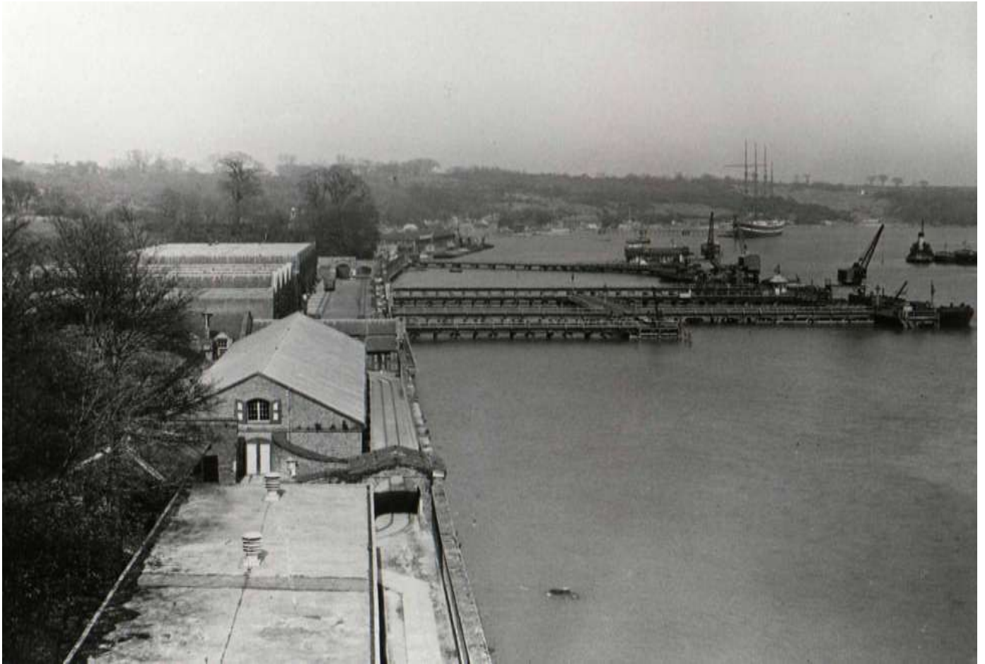
Figure 49. Looking downriver and to the north and probably photographed from an upper window of Upnor Castle. The view shows in the immediate foreground the Laboratory Sheds (with concrete flat roofs added in WW2), to the left the Shifting House with its 19 th century curved walls, and adjacent alongside the wharf the No. 1 Shell Store. Beyond you can see 'A' Magazine, 'and B' Magazine (Evans 2000b: 63)
