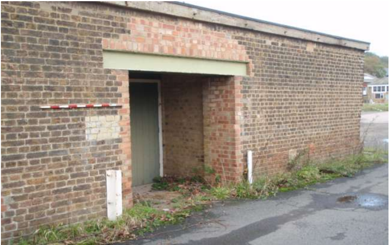
Plates 35, 36. Small Arms Store showing rebuilt main entrance and (below) window- 1m scale
