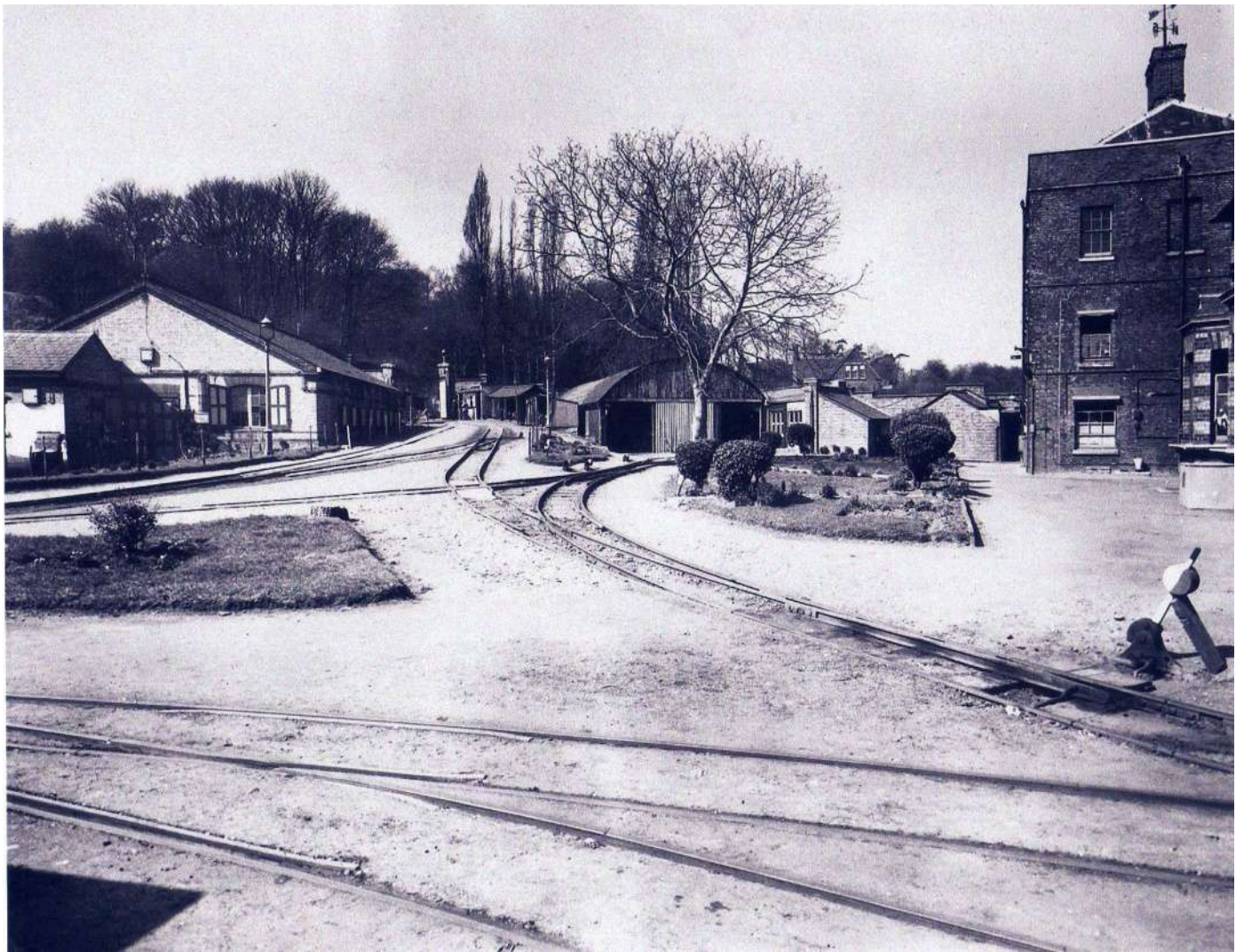
Figure 48. This photograph shows the former civilian houses (right), the Truck Shed (centre), and to the right the Latrine Block. To the left of the Truck Shed across the railway tracks can be seen the Wet Guncotton Store and Mine Testing Room (Evans 2000b: 67)
