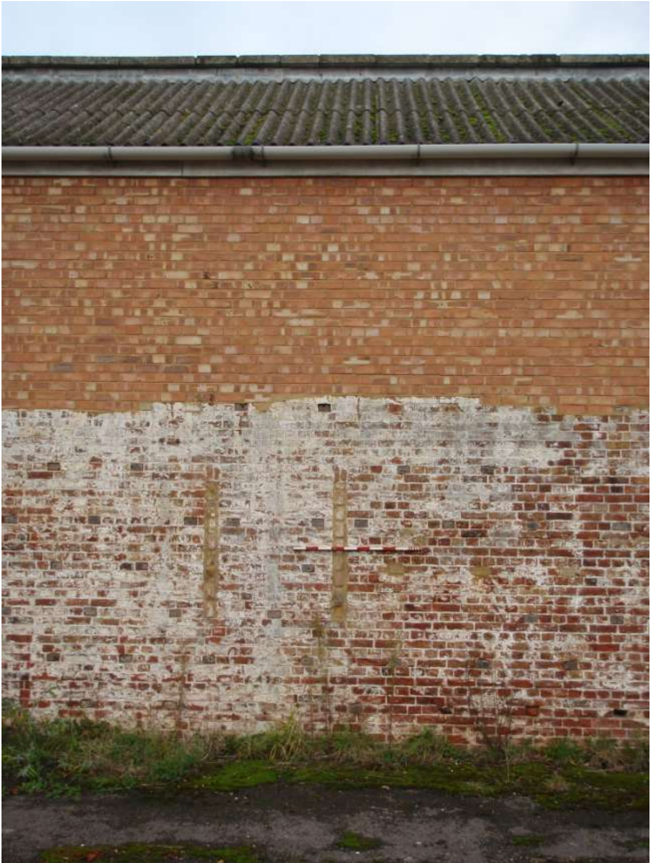
Plate 55. Detail of hardwood blocks, ventilation slots, and repaired wall- 1m scale
