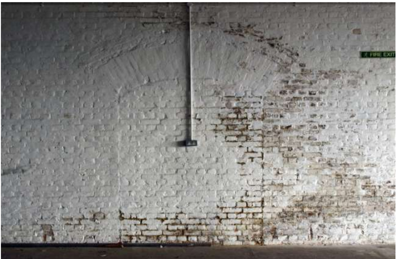
Plates 66. 67. Internal view looking south to blocked up entrance to Magazine 'A' and (below) detail
