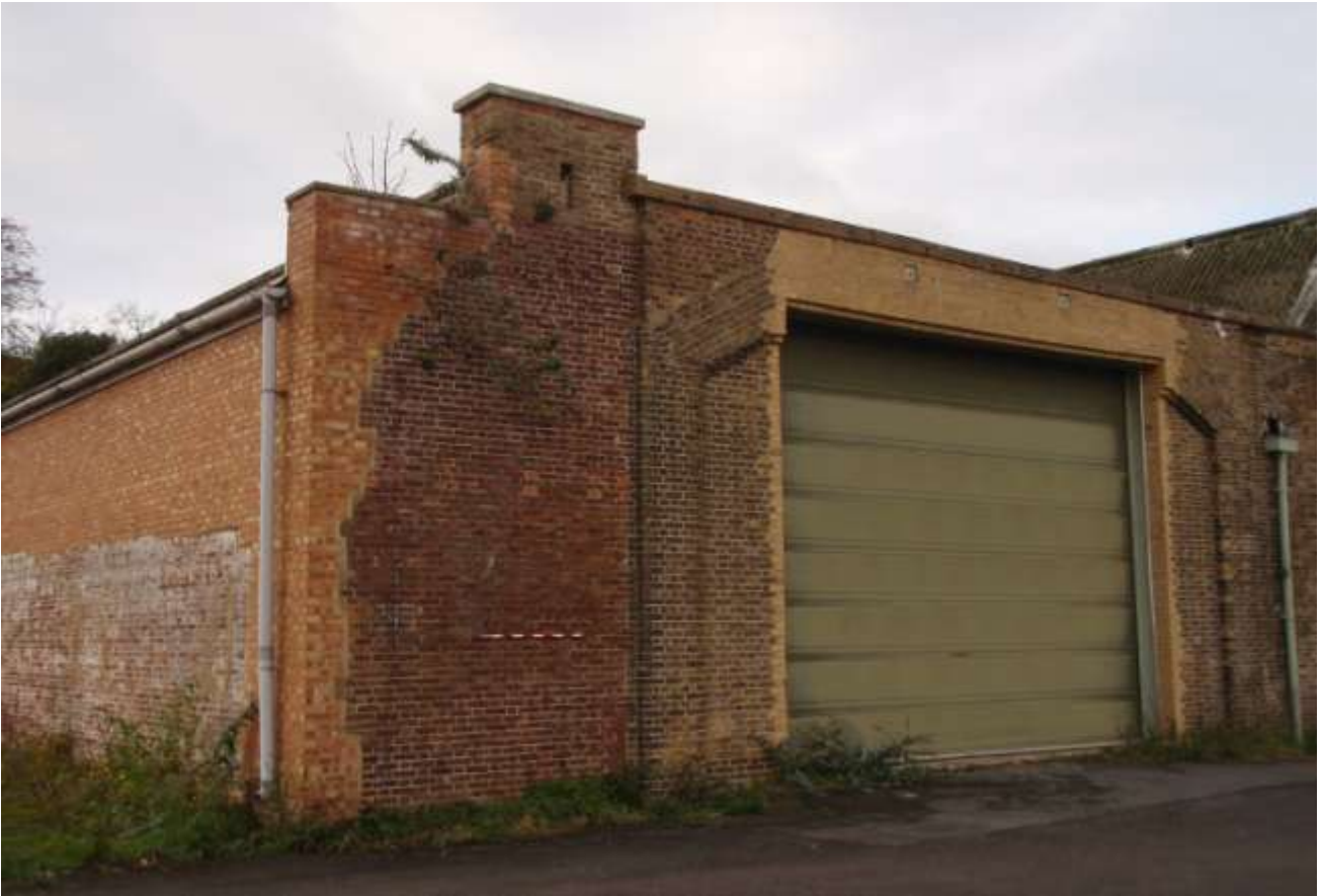
Plates 56. 57. View of front of the Empty Case Store showing four phases of build, and (below) rear view
