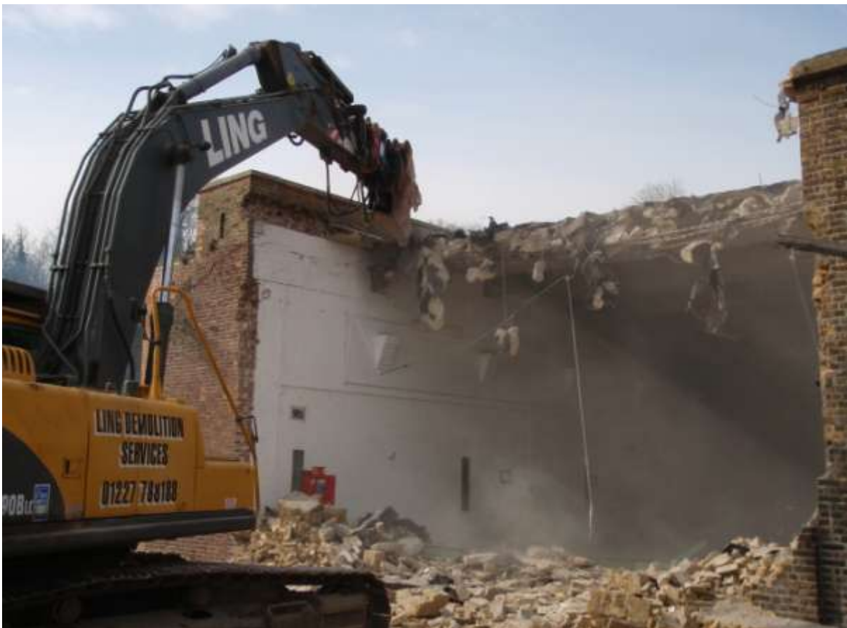
Plate 78. Demolition of the reinforced roof of the Empty Case Store
